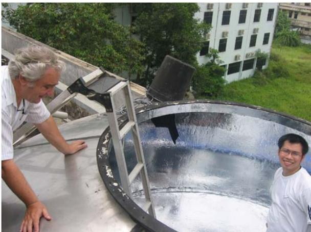
Dong coating the wall of the large tank with aluminized mylar
