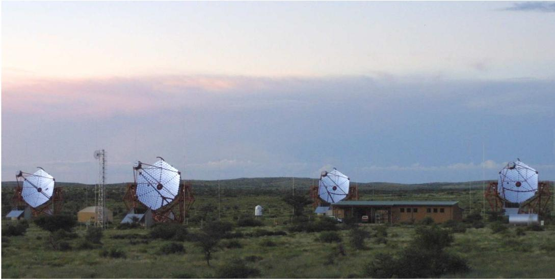
Figure 9: The High Energy Stereoscopic System (HESS, Namibia) includes four telescopes at the corners of a  $120 \times 120 \text{ m}^2$  square, operating above 100 GeV. Its field of view is  $5^\circ$  and its resolution a few arc minutes. To take a picture of the Crab takes only 30 seconds.
