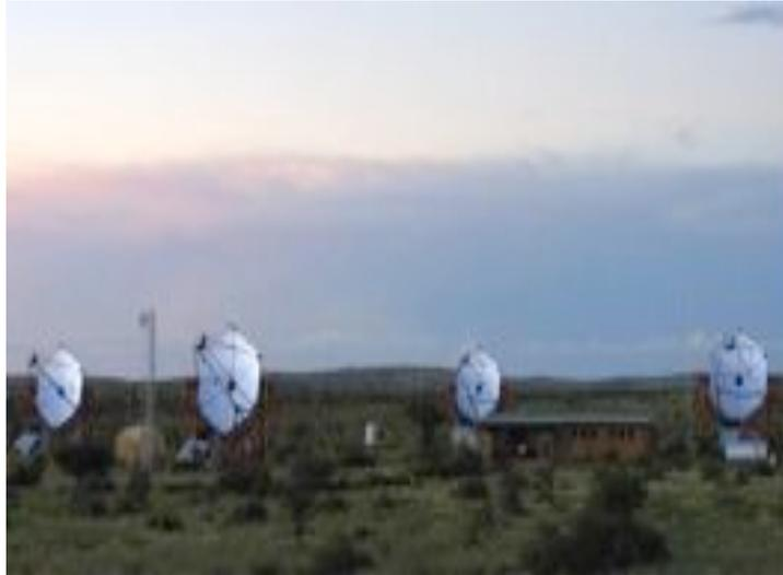
**Figure 1.3:** The High Energy Stereoscopic System (HESS, Namibia) [11] includes four telescopes at the corners of a  $120 \times 120 \text{ m}^2$  square, operating above 100 GeV. Its field of view is  $5^\circ$  and its resolution a few arc minutes. To take a picture of the Crab takes only 30 seconds.
