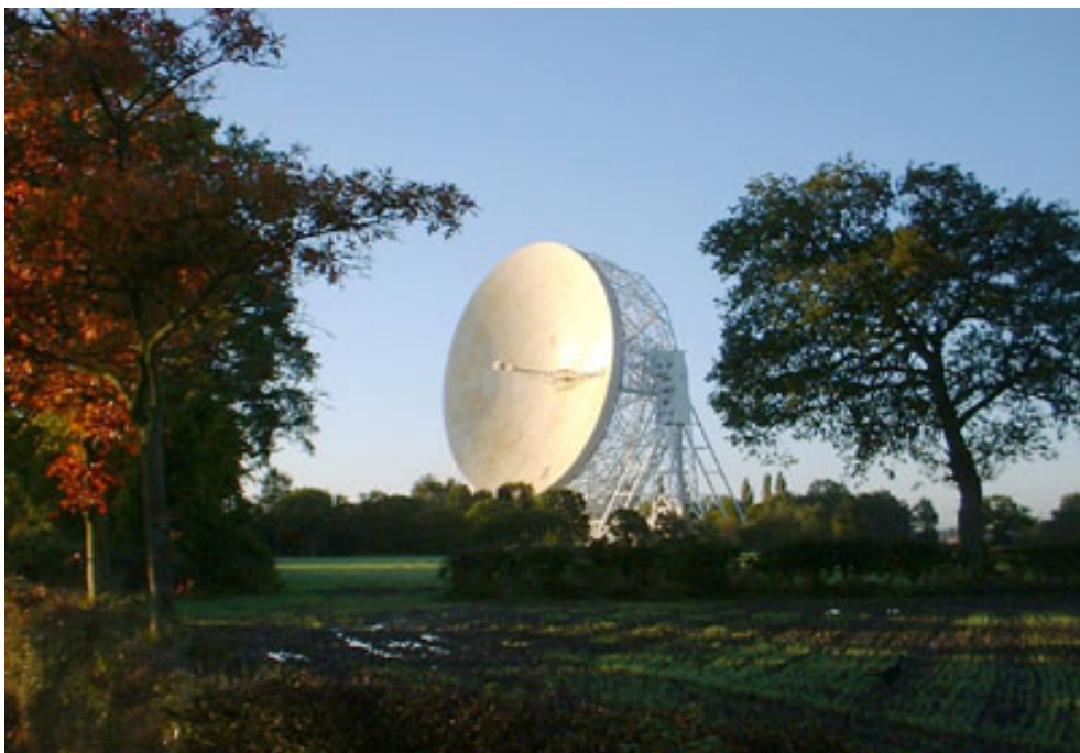
Figure 2.2 The Jodrell Bank antenna in the United Kingdom is 75 m in diameter.
